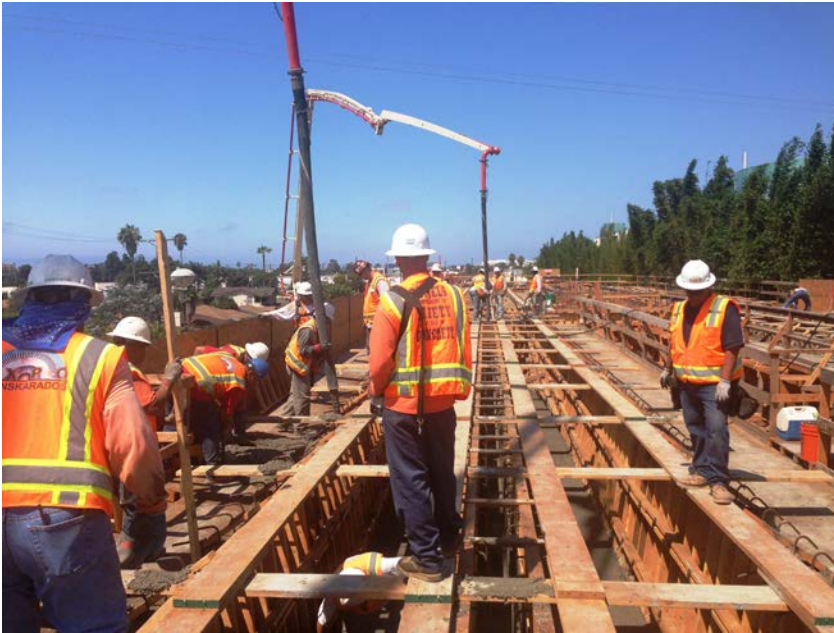
Top and Center: Work crews pouring concrete for Bundy Bridge
