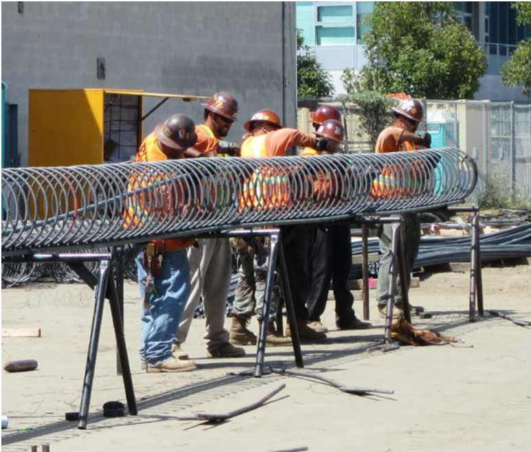
Top: Work crew assembling rebar cages
