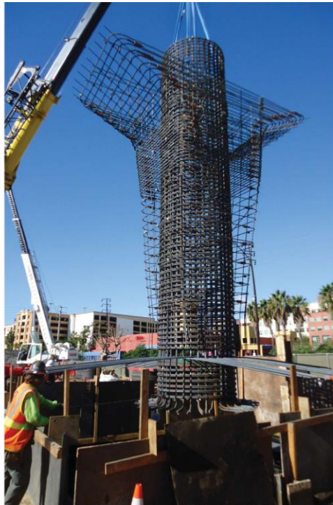
Setting Bent 3 Column Cage at Olympic Bridge_DSC01110
