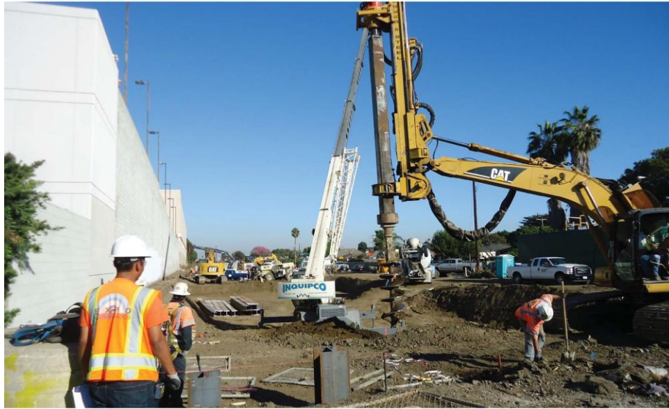
Drilling and Setting Shoring Beams at Bundy_DSC01062
