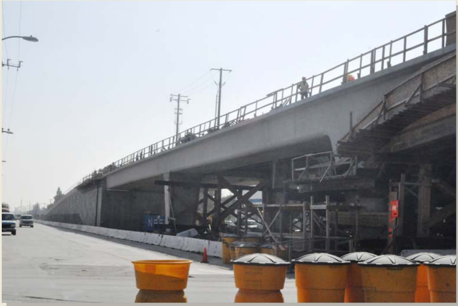
Falsework Removal at La Brea Aerial Structure
