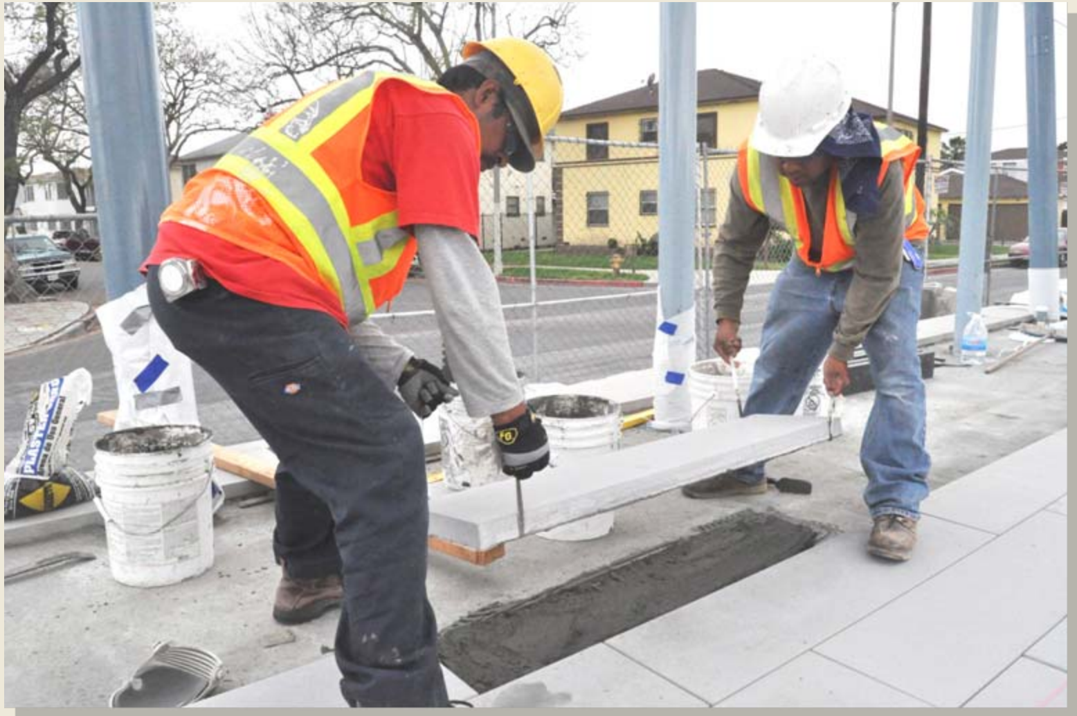
Tile installation at the Crenshaw Boulevard Station
