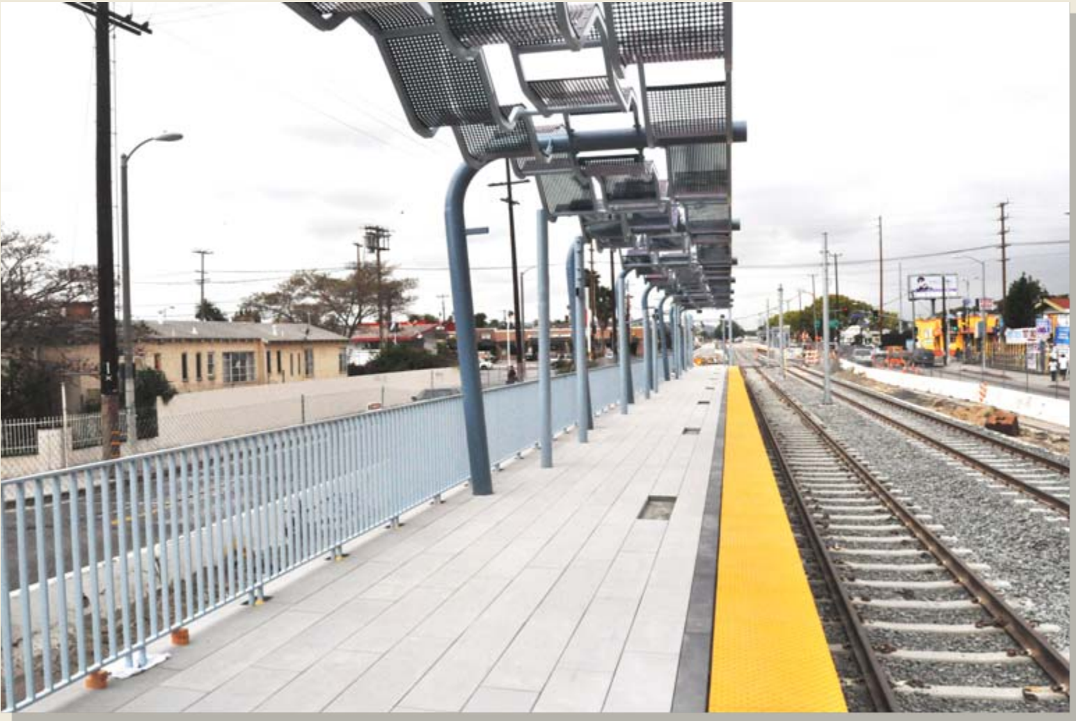
Western Avenue Station with installed canopies, fencing and tiling
