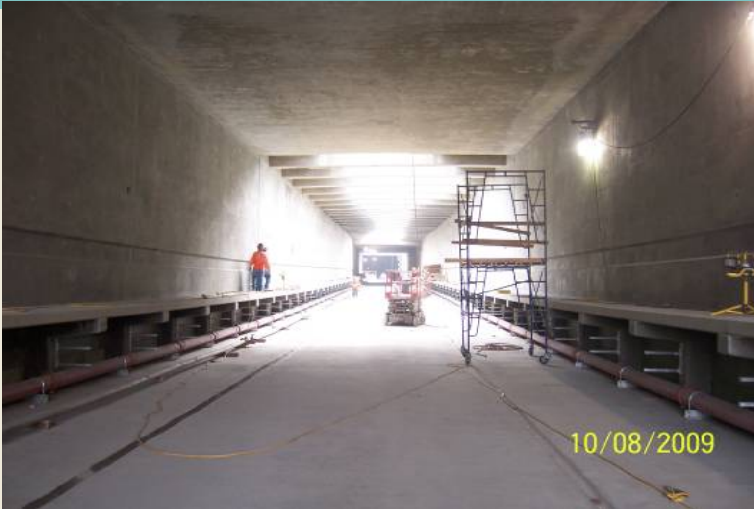
Walkways and Wet Stand-Pipe Installation at Grade Separation Trench Structure
