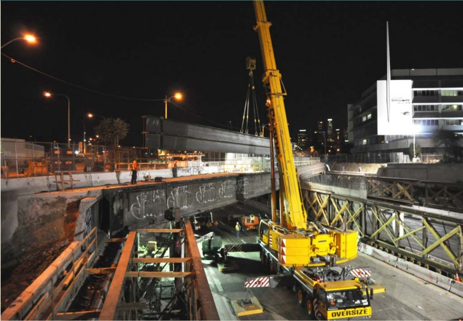
Girder Installation at I-110 Flower Street Overcrossing
