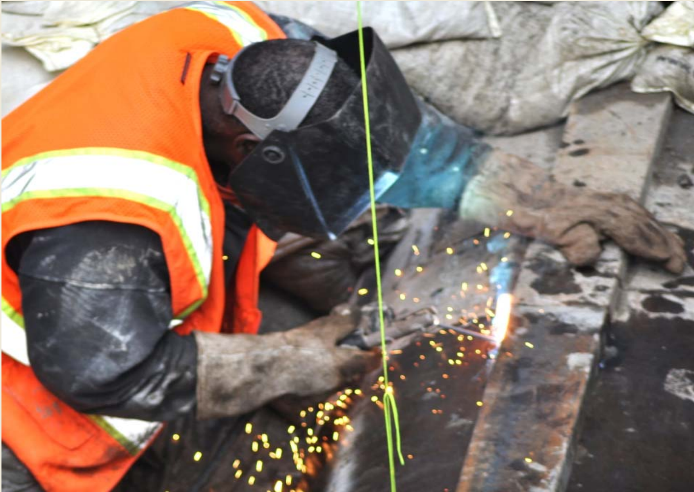
Electrical Vault Welding at Crenshaw
