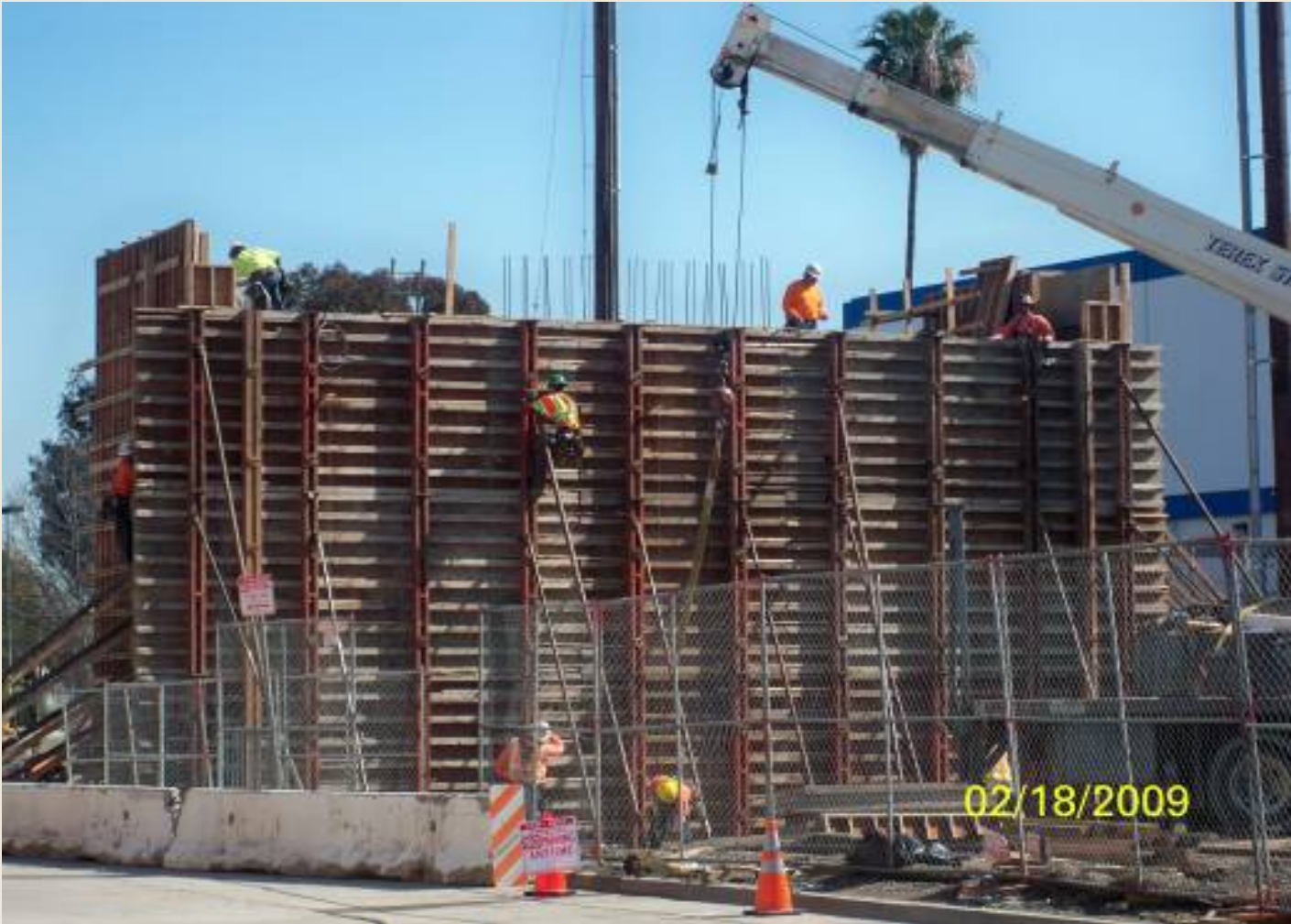
Rebar Installation at La Brea Overcrossing Structure, Abutment No. 1
