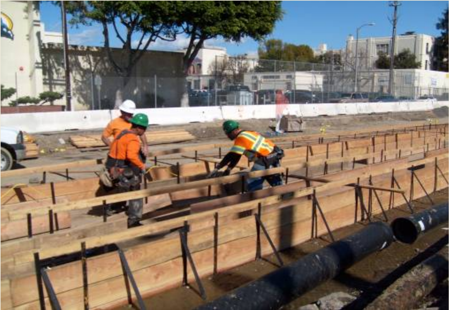
Placement of Foundation Forms for Western Avenue Station
