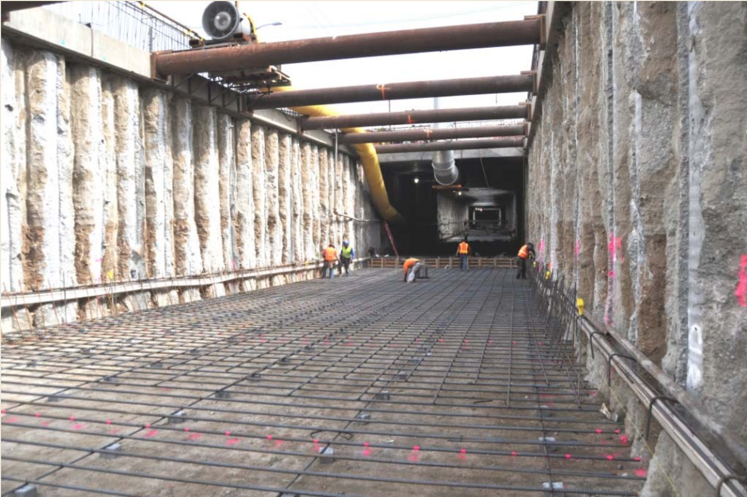
Rebar Installation for Slab Placement at Trench Structure
