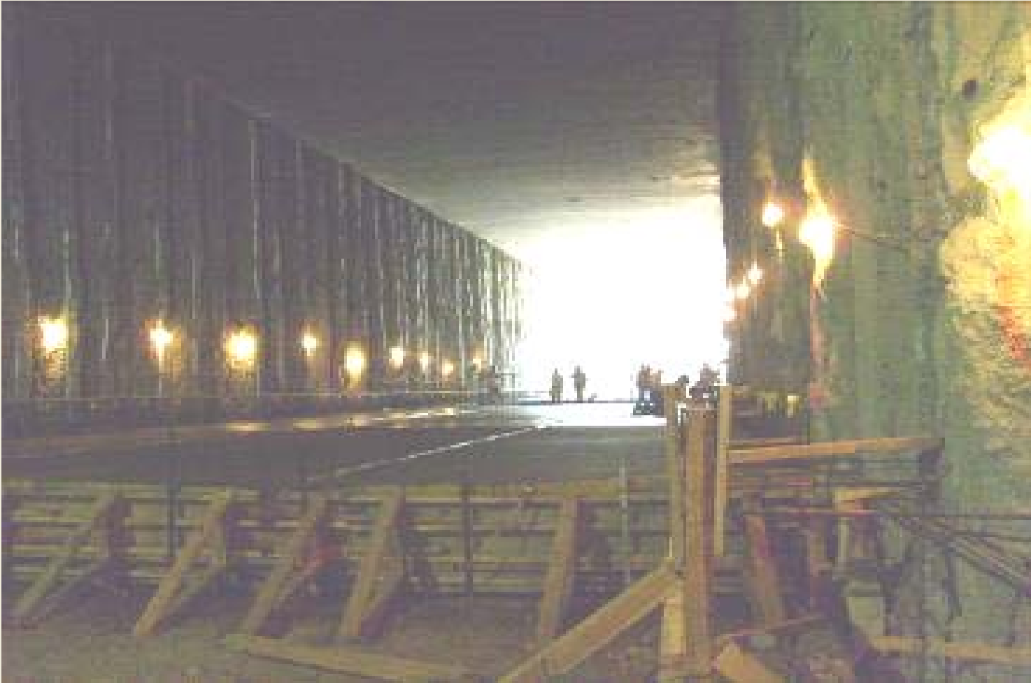
Slab Placement and Wall Rebar Installation at Trench Structure
