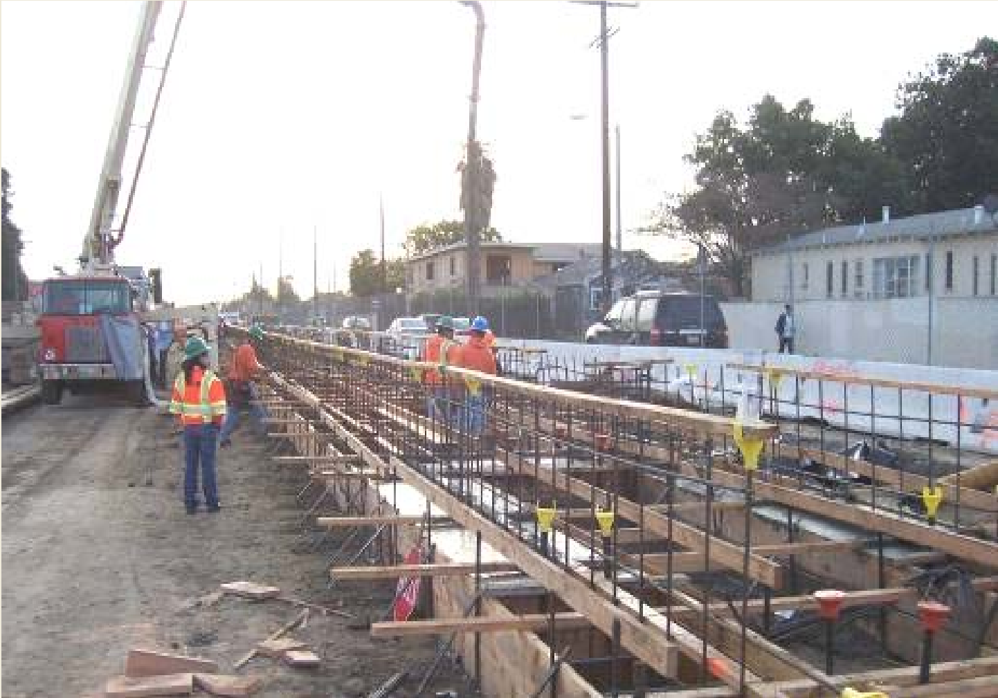
Concrete Placement for Western Avenue Station— East Platform Footings
