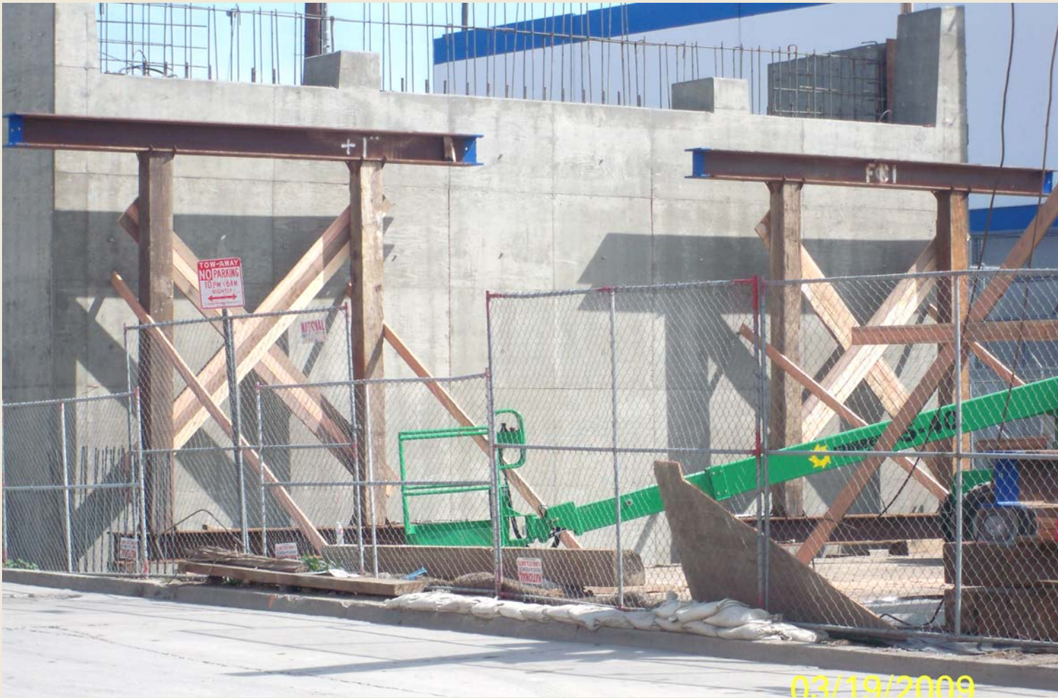
Erection of Falsework for La Brea Overcrossing Structure
