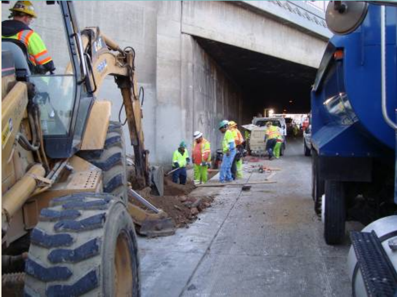
Demolition of Shoulder Along Southbound I-110 Freeway
