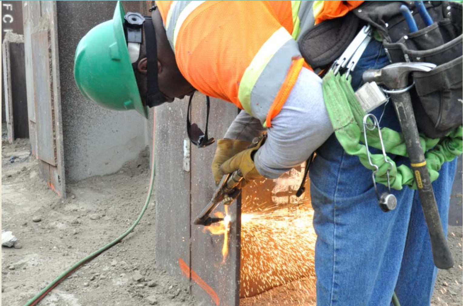
Removal of Shoring at National Boulevard
