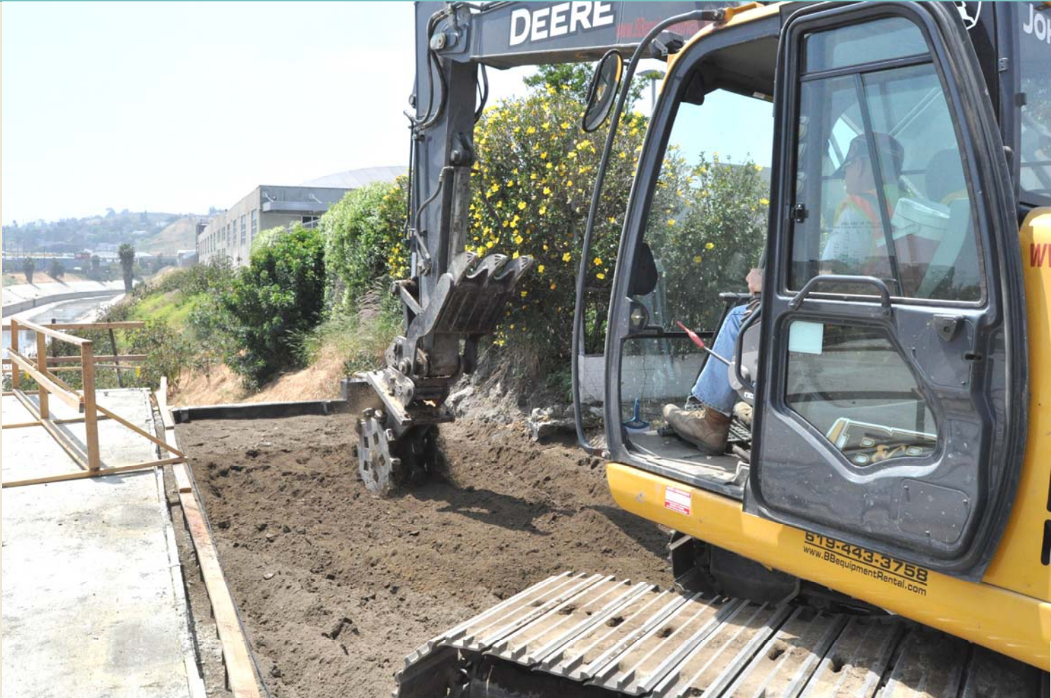
Structural Backfill for West Side of National Boulevard Bridge
